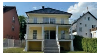
Villa in Schwetzingen
